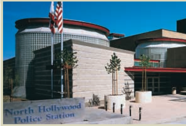
North Hollywood Police Station, N. Hollywood, CA // Architect: Meyer & Allen Associates ARGUS® Pattern and HEDRON® Corner Block
